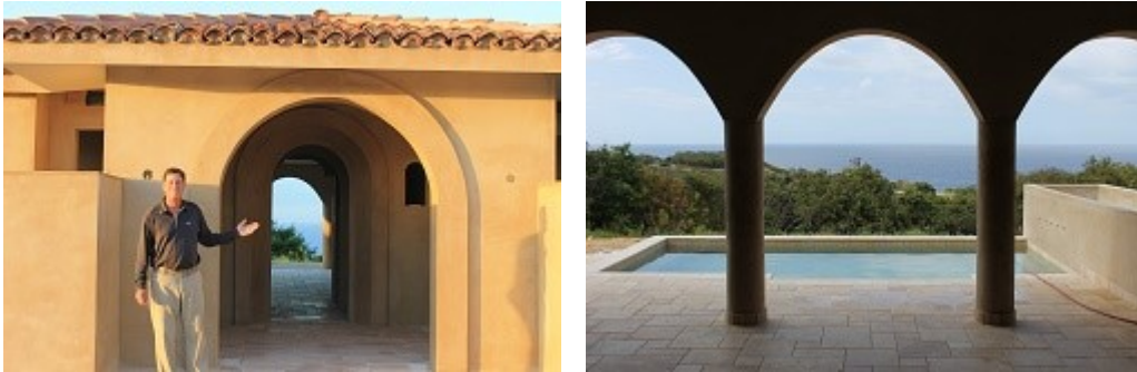
Left: Stanley Pasarell, co-owner of Royal Isabela, in front of a soon-to-be-completed Fairway Villa. Right: The view from a Fairway Villa, under construction, at Royal Isabela.
